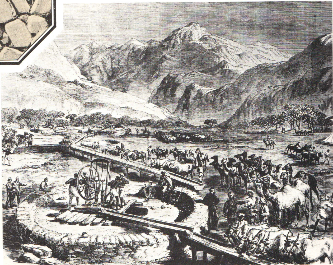
Draught-bullocks slake a thirst at Kumayli's wells. The water was pumped to the surface through metal tubes sunk deep in the earth.
